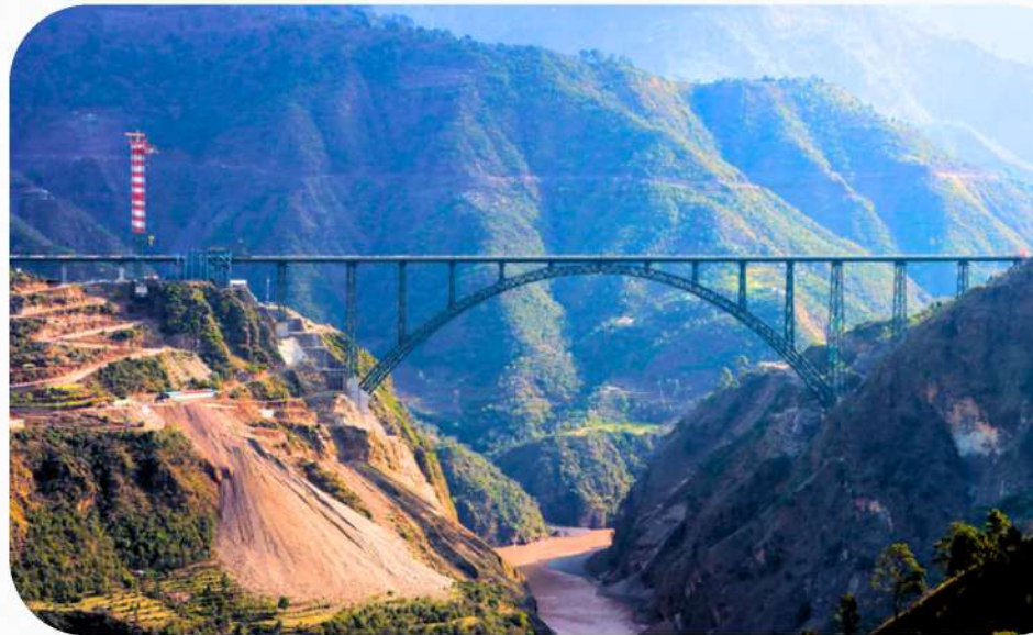
Chenab Bridge, Jammu & Kashmir, India
