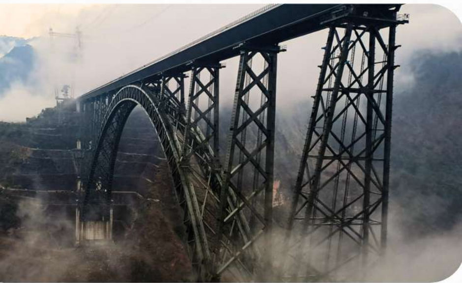
Chenab Bridge, Jammu & Kashmir, India
