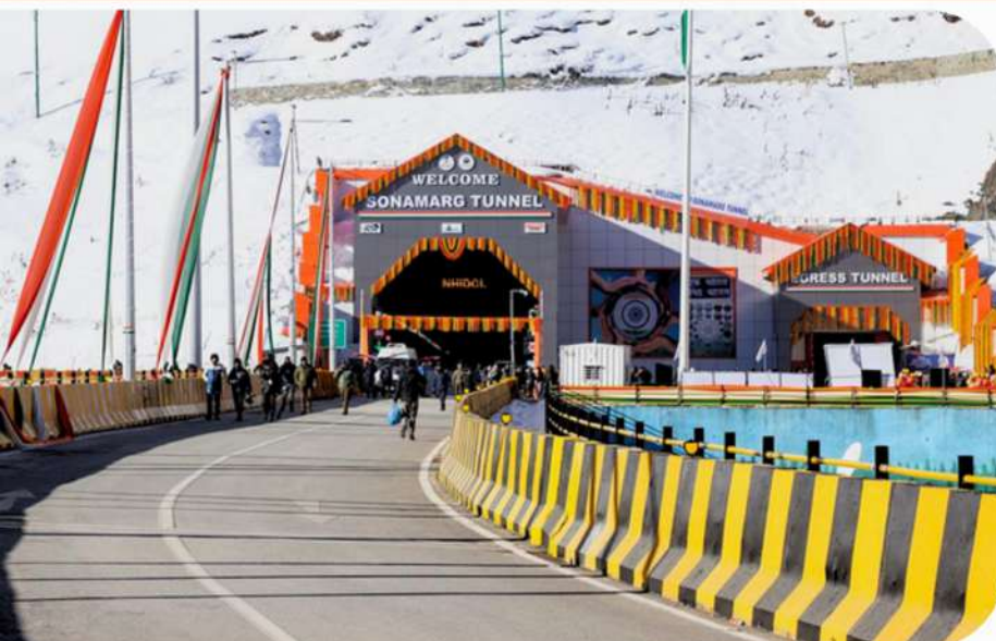
Sonamarg Tunnel (Z-Morh tunnel), Jammu & Kashmir, India
